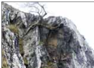
Cliff on the fault-line: new rock-fall, probably caused by tree growth
