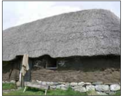
Reconstruction of a large turf house
