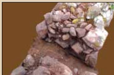
This cross-section shows the outer and inner facings made of large stones, infilled with smaller stones
